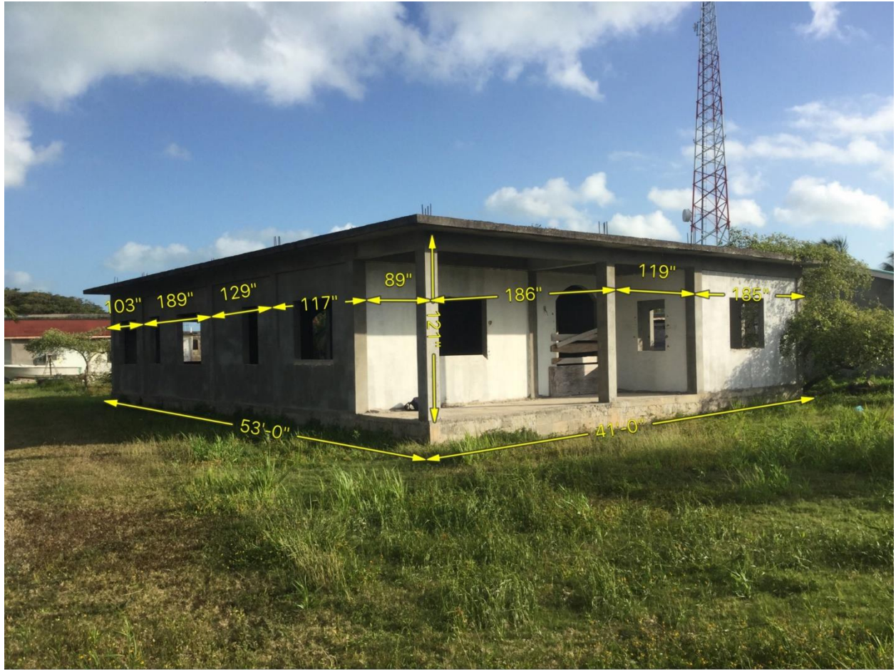
PARCEL NO. 329, LOOKING TOWARDS THE WEST
